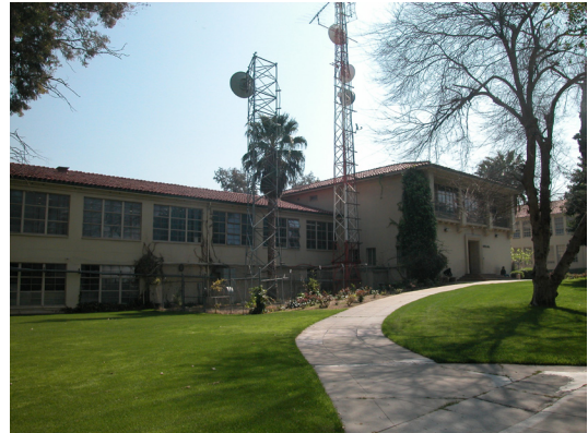
North Hall Building - To be Demolished
