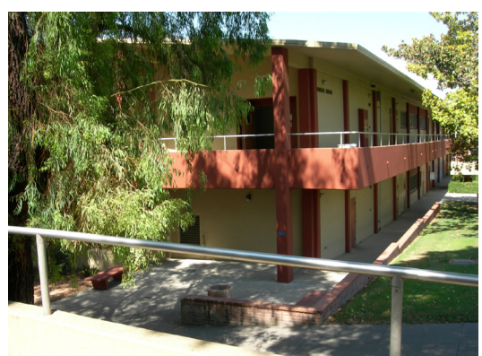
Physical Science Building - To be Demolished
