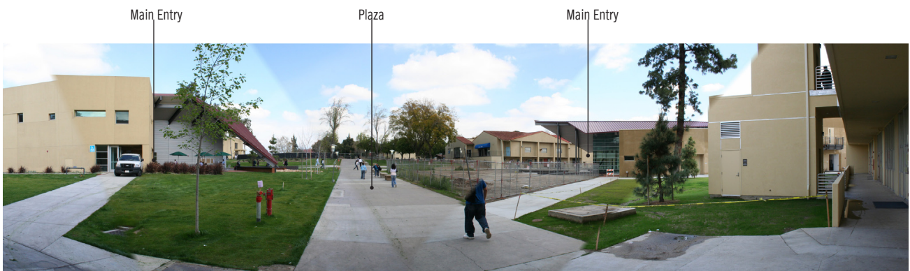
View from Business building
