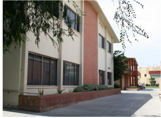
Chemistry Building - To be Demolished
