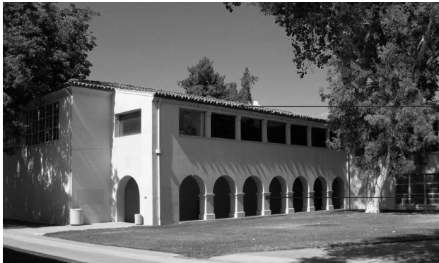
North Hall - To be demolished
