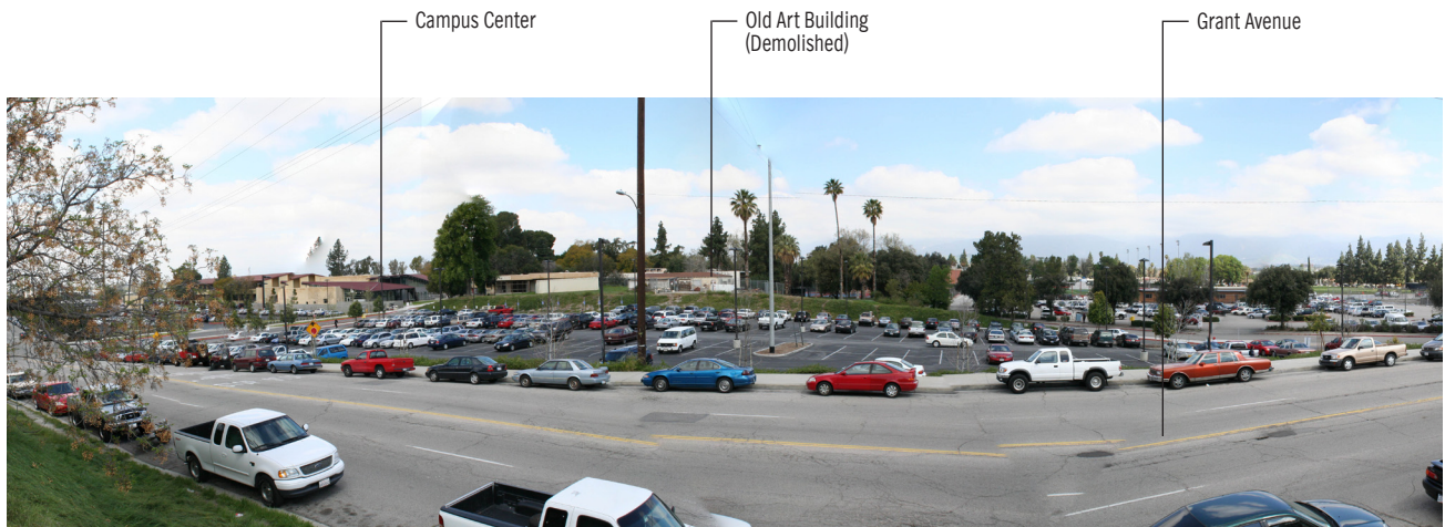
View of Grant Avenue looking into campus.
