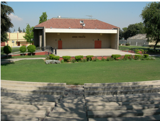
Planetarium - Recommended for Demolition.
